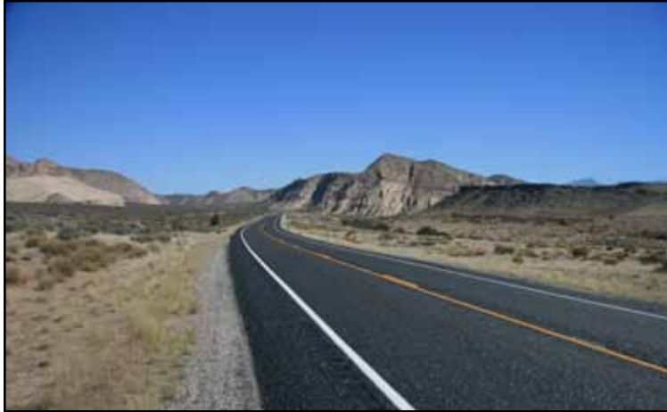
Above: Highway 18 was rumblestripped by UDOT in a manner that appears to against their own guidelines. The rumblestrip is just to the left of the white fogline and leaves little room for cyclists to ride on the shoulder. Photo: Bryce Pratt
