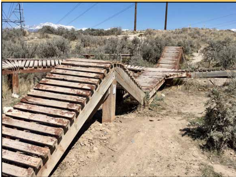
This bridge at Eagle Mountain may be wide, but adding elevation makes it more challenging. Photo by Tom Jow
